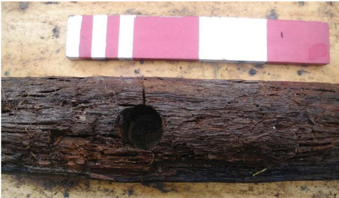
Plate 24: Detail of dowel hole in Timber 63. Scale 0.20 m
